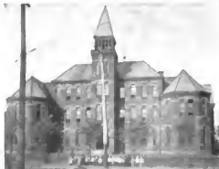
CENTRAL SCHOOL BUILDING, WELLSVILLE
